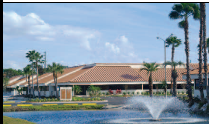
Meridian Gateway Center Four Buildings totaling 165,013 sf, Flex Warehouse, St. Petersburg, Florida 5,500 - 41,000 sf available for lease www.MGCpinellas.com
