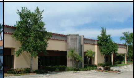
Meridian Concourse Center Four Buildings totaling 217,382 sf, Office, Flex Warehouse, Clearwater, Florida 5,000 - 6,000 sf available for lease
